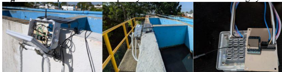
Figure 2. Components and temporary installation of the monitoring system
